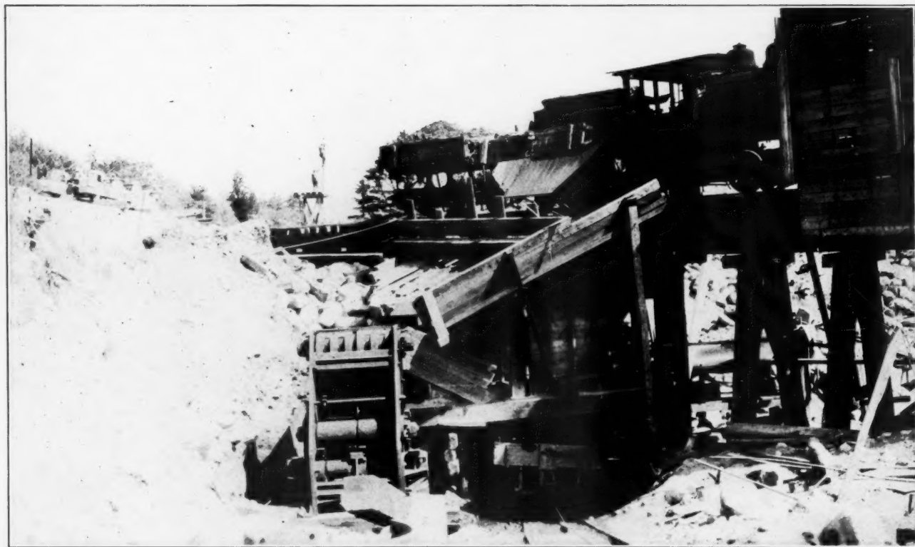
Upper Left—Sand settling tank and also a sand bin of small capacity receiving sand delivered by bucket elevator which takes product of dewatering screw conveyor. Upper Right—Conveyor belt used for loading freight cars. Lower—Cars from the pit being dumped into grizzly over the new crusher. Note car under hopper which carries material up to the plant.
